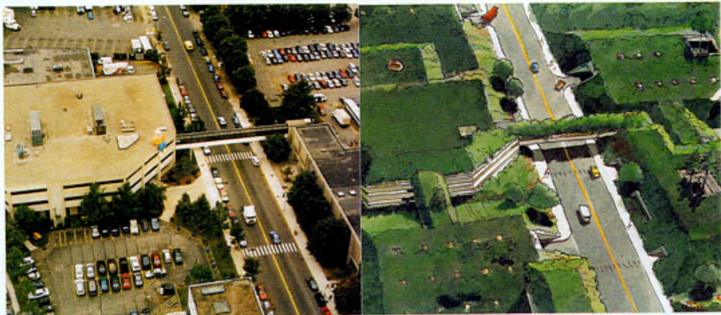
Architect Malcolm Wells would like to green this Boston television station and its parking lots (left) by putting them underground (right).
