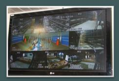
The security system of the facility includes Closed Circuit TV to monitor entry / exit areas, the lobby and inside the garage. High resolution digital IP cameras take two photos of each car on entry
