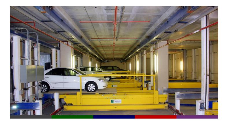
Robotic Parking Systems has successfully completed throughput testing of its recently completed 2,350 capacity Al Jahra Court Automatic Parking System in Kuwait. TÜV Nord certified a peak traffic throughput capacity of 425 cars per hour. Throughput capacity is the total number of cars per hour that can be handled in a combination of inbound and outbound vehicle traffic.
