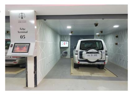
The driver parks the car on its own pallet in the entry / exit terminal, and the car is never touched by machines or humans as it is moved. This eliminates any problems with parking cars that are low to the ground as well as the typical dings and dents that occur in parking lots or concrete ramp garages. Cars are stored in a fully enclosed building and are 100% secure from theft of the car or its contents as well as vandalism.
