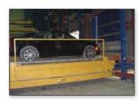
8. The Robotic Parking Systems' machinery delivers the car facing forward so that it is safe and easy to exit the garage.
