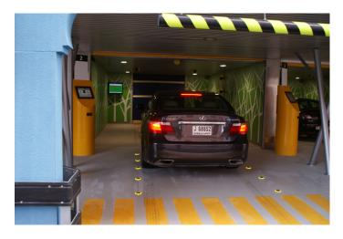
When the owner of the car returns to the ground floor exit at the Ibn Battuta car park, he or she goes to a kiosk and follows the simple instructions before swiping his card again. The system informs the car owner on flatbed screens which gate to go to for the car. Retrieval by the system takes approximately 1 to 2.5 minutes on average, with the car then ready to drive away.
