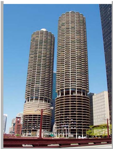
Parking for the structure is likewise self-contained: The lower third of the 65-story towers is a continuous up-spiral parking garage with space for 896 vehicles each.
